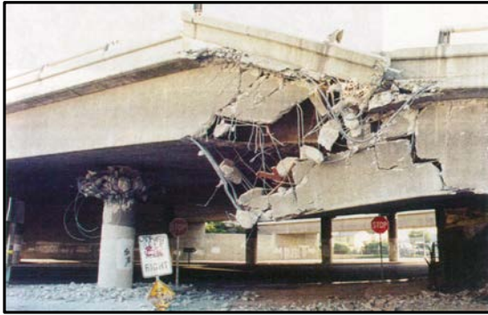
La Cienega-Venice Blvd Undercrossing
