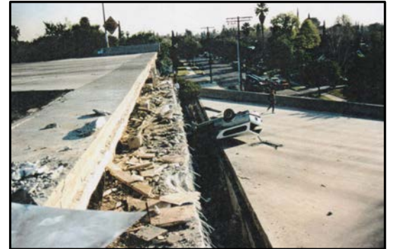
Mission Gothic Undercrossing
