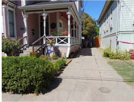
Topped “cripple wall”
