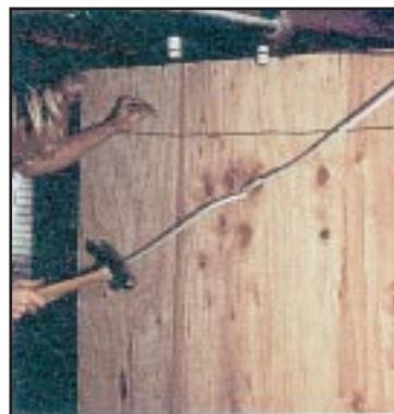
**Sheets of plywood** nailed to the cripple walls help to prevent damage from shaking in this weak area of your house. Cross-bracing within the framing is not enough.
