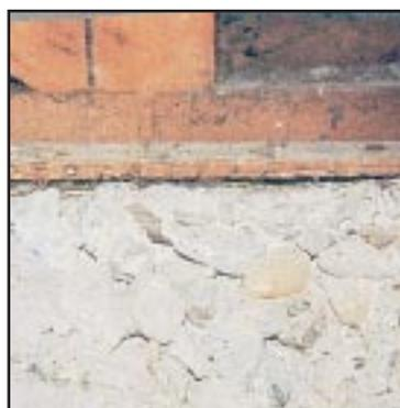
**Faulty materials** such as rotten wood and porous concrete should be replaced. Risky conditions in concrete include cracks wider than one-eighth inch, large voids, or "honeycomb" concrete. If the concrete chips or flakes when you poke it with a screwdriver, it may be unsafe. **NOTE:** If you suspect faulty material, you may need the assistance of a licensed engineer or architect to design a solution.
