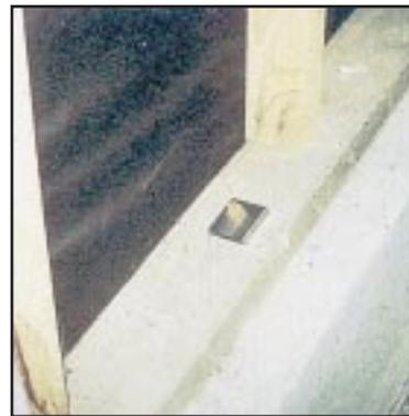
**Bolts** secure your home's mud sill to the concrete foundation. The mud sill should be anchored as specified on the Department's Standard Plan.
