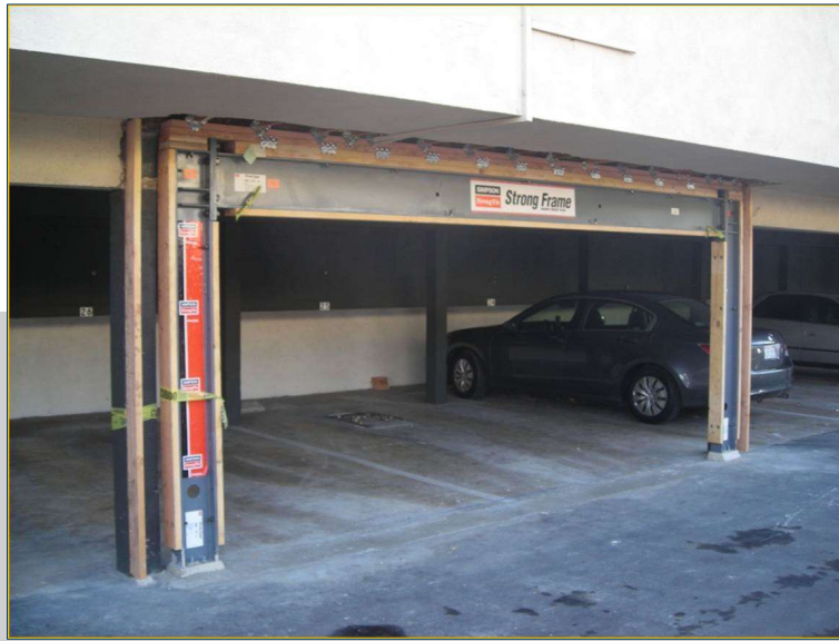
Steel frame around garage door opening
