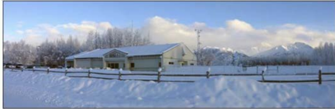
National Tsunami Warning Center, Palmer, Alaska in 2021
