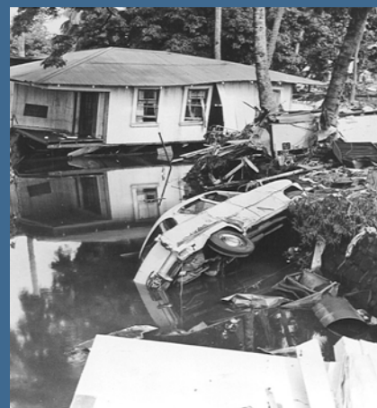
May 22, 1960, M9.5 Chile EQ Damage in Hilo, Hawaii
