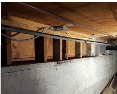
Crawlspace Before Retrofit
