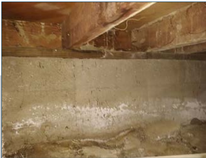
Crawlspace Before Retrofit
