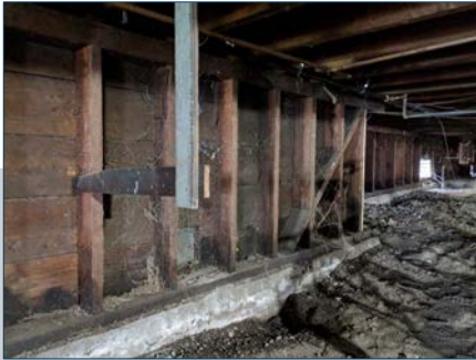
Crawlspace Before Retrofit
